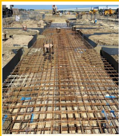
Central foundation reinforcement complete and concrete pour in progress.
