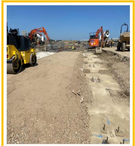
Building MEWP mat installation in progress.
