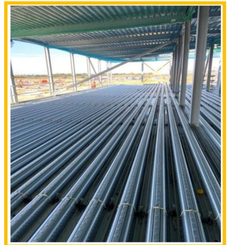
Metal decking and shear studs complete to 2 nd floor.
