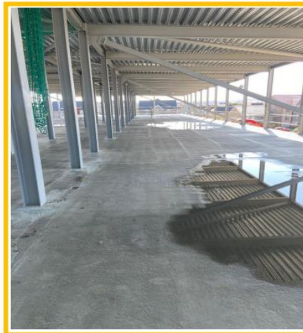
2 nd floor slab first section poured.
