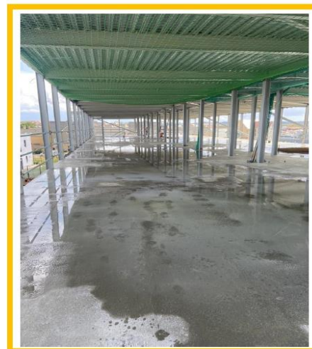
2 nd floor slab fully poured and complete.
